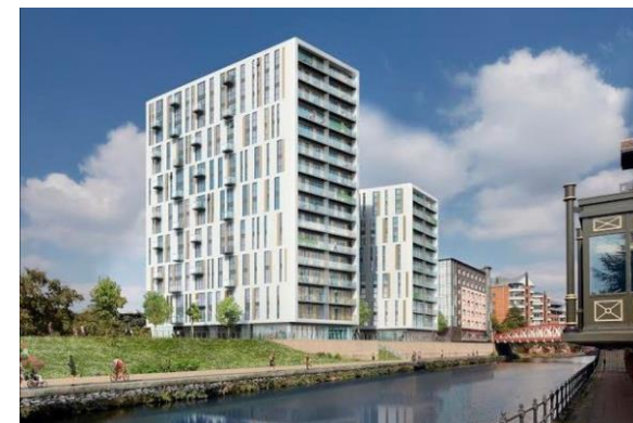
The Slate Yard, Salford
